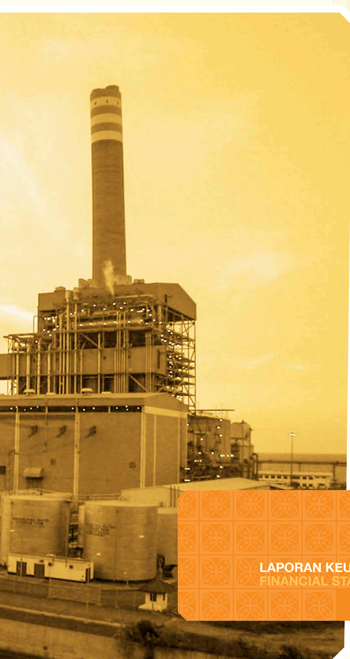
Pembangkit Listrik Tenaga Uap Paiton Jawa Timur, Indonesia Steam Turbine Power Plant Paiton East Java, Indonesia
